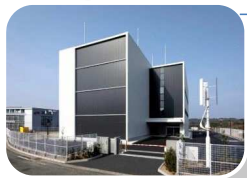
Okayama Data Center
