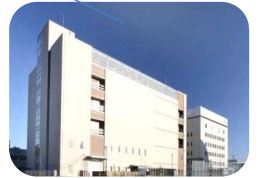
Shizuoka Data Center 12
