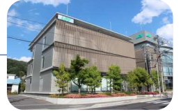
LCV Data Center
